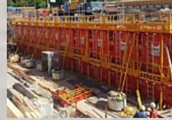
Chantier rond-point SERRA
