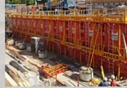
Chantier rond-point SERRA
