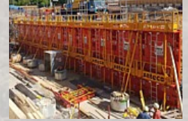
Chantier rond-point SERRA
